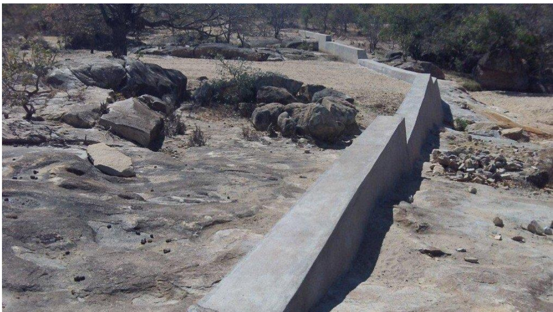
Figure:5 Rainwater harvesting - a sand dam in Gwanda district, Zimbabwe
